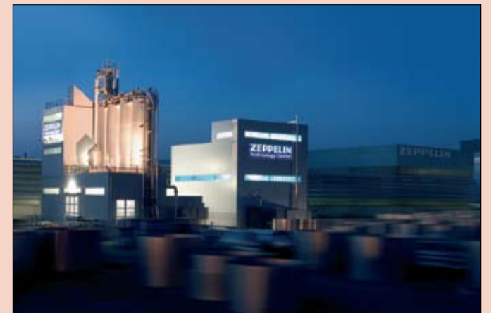
Zeppelin's Friedrichshafen test centre by night; here at least one world first in pneumatic conveying technology is reported to have been pioneered.
