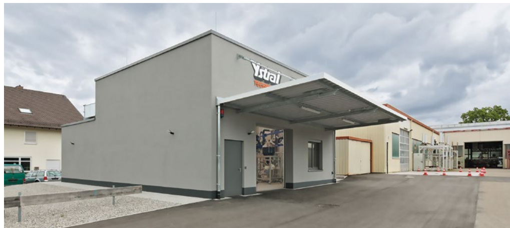
The new trial centre was constructed in a compact cubic design on an area of around 150 m 2 and can be expanded with an additional trial building
