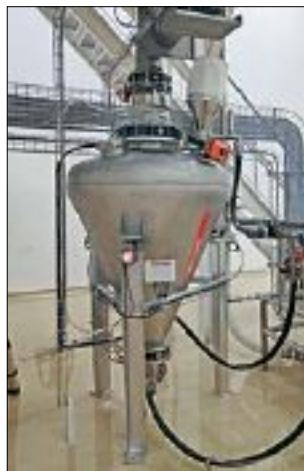
The Gericke Pulseflow pneumatic conveying sender for salt.
