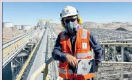
The cement plant in Arequipa, Peru.
